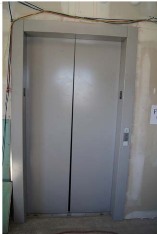
Door Jamb After FB4-DEN67 (functional)
