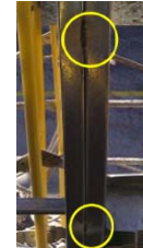
Welding of double studs
