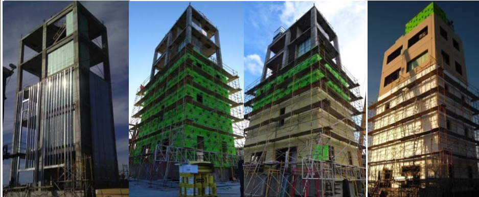
Metal "balloon framed" studs
