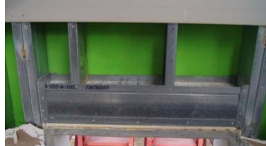
Box header above opening
