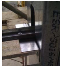
Clip connection between vertical and horizontal studs
