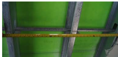
Vertical studs spacing @ 16"
