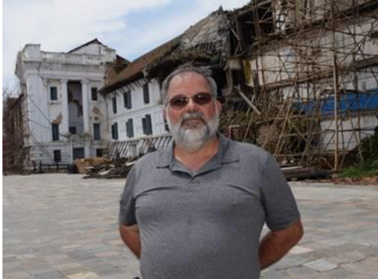
Speaker next to building damaged by the April 2015 Gorkha (Nepal) Earthquake
